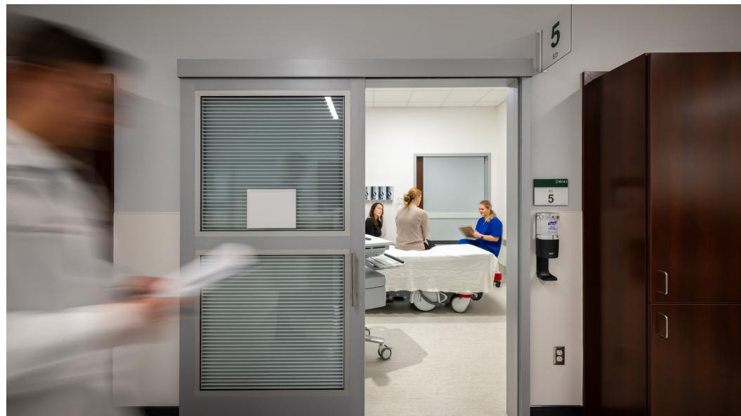
WHERE A SWING DOOR COULD HAVE DEMANDED UP TO 30 SQUARE FEET OF CLEARANCE, EXAMSLIDE GLIDES SMOOTHLY ALONG THE WALL FROM A TOP-HUNG TRACK.
