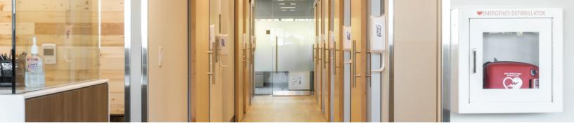
Finally, AD Systems' ExamSlide hardware is ADA compliant, so all patients can have equal access to PacMed's care. Further, because sliding doors do not need approach clearance and are fitted with soft closers, they are easily operated by all. This both embodies PacMed's commitment to putting patient needs first and the design goal for a building that supports positive occupant experiences.
